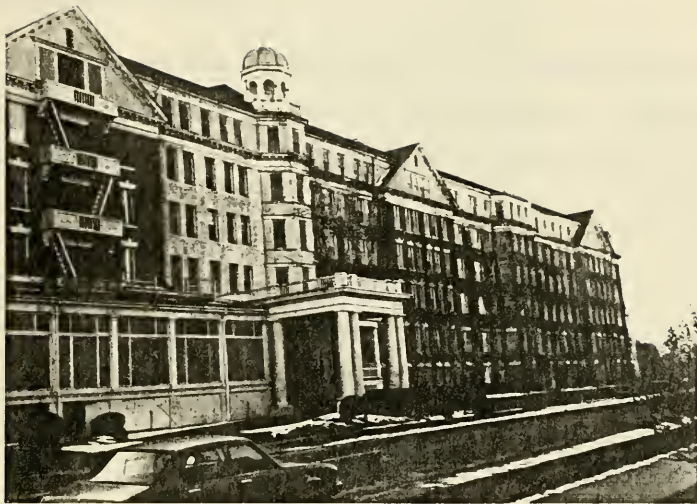
Plate 27: North Wing, North Elevation, 1985
